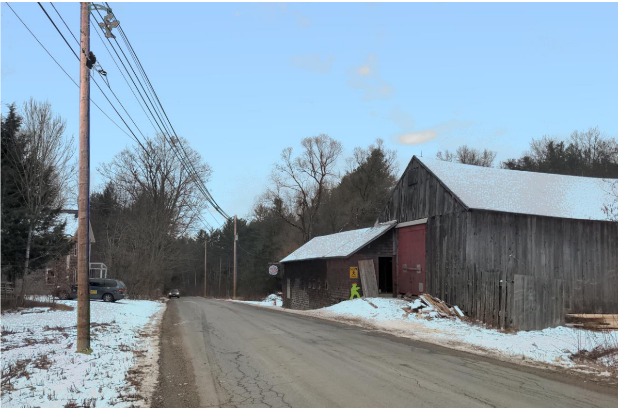
Photo #2-B: View of proposed structure P-28 on the left and looking towards proposed structures P-27 and P-26
